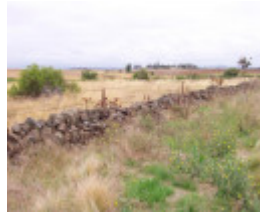
Dry Stone Wall P298
