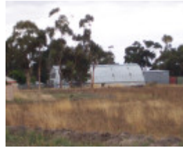
Former Radio Station
