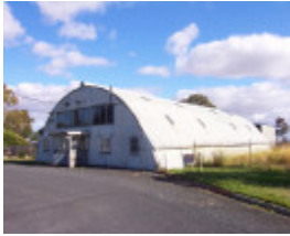
Former Army Radio Station
