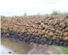
Holden Road Dam
