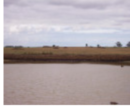
Holden Road Dam
