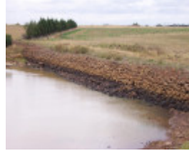
Holden Road Dam
