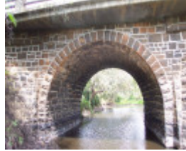
Bridge over the Kororoit Creek
