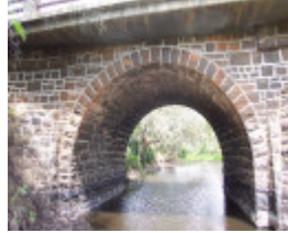
Bridge over the Kororoit Creek
