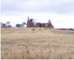
Mount Aitken site and ruin
