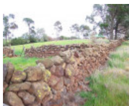
Dry Stone Wall A272
