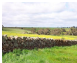
Dry Stone Wall A274
