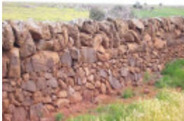
Dry Stone Wall A277
