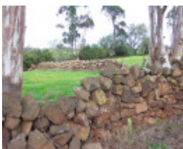
Dry Stone Wall A273
