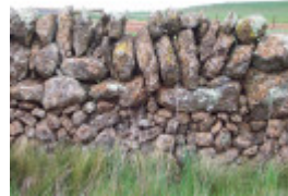
Dry Stone Wall A277
