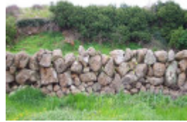
Dry Stone Wall A276
