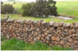
Dry Stone Wall A275
