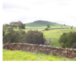
Dry Stone Wall A275
