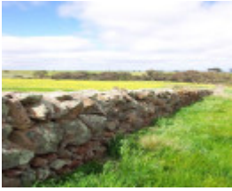
Dry Stone Wall A274
