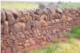
Dry Stone Wall A277
