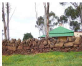
Dry Stone Wall A272
