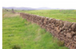
Dry Stone Wall A277
