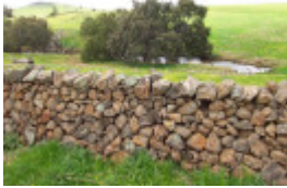
Dry Stone Wall A275
