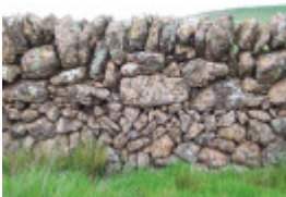
Dry Stone Wall A277
