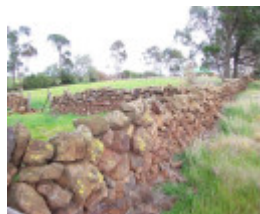
Dry Stone Wall A272
