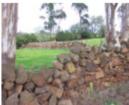
Dry Stone Wall A273
