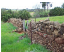
Dry Stone Wall A273
