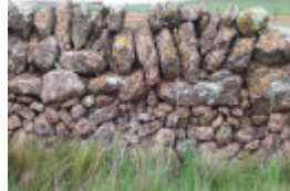
Dry Stone Wall A277
