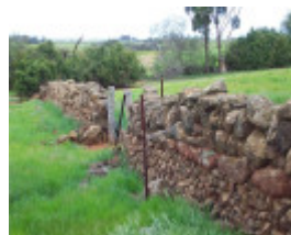
Dry Stone Wall A273
