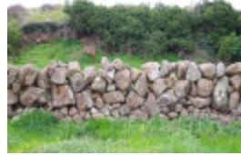
Dry Stone Wall A276
