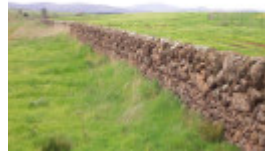
Dry Stone Wall A277
