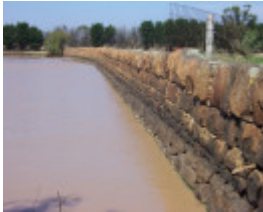
The Plumpton Dam
