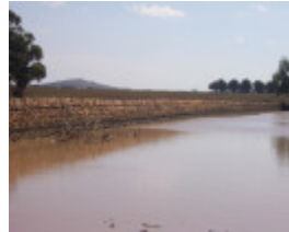
The Plumpton Dam
