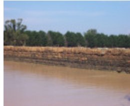
The Plumpton Dam
