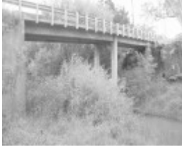
Bridge Road bridge over the Toolern Creek
