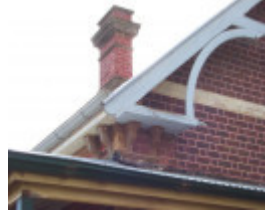
Kippenross - eave detail
