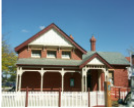
Former Melton Courthouse
