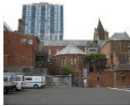
Francis Ormond Bldg_Melbourne_rear view_8 Jan 2008
