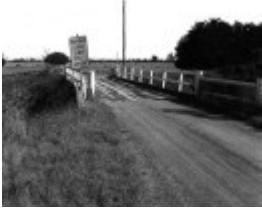
Swamp Bridges & Swamp Drains
