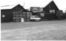
Towts Cool Store & Packing Shed
