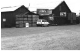
Towts Cool Store & Packing Shed
