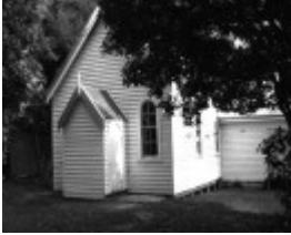
Tynong North Methodist Church - Former Christ Church
