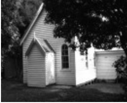
Tynong North Methodist Church - Former Christ Church
