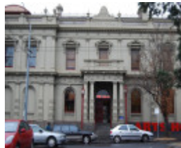
3016 Hotham Town Hall Queensberry St Entrance 02
