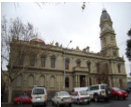
3016 Hotham Town Hall Queensberry St View 02
