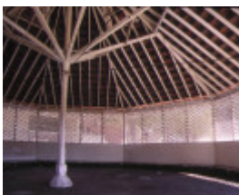
infant building & shelter shed coburg primary school no 484 bell street coburg interior of shelter feb 98
