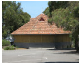
INFANT BUILDING AND SHELTER SHED, PRIMARY SCHOOL NO.484 SOHE 2008
