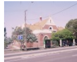
1 infant building & shelter shed coburg primary school no 484 bell street coburg front view feb 98
