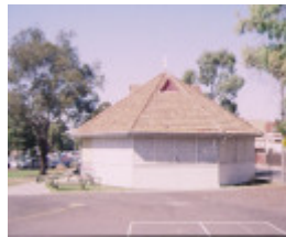
infant building & shelter shed coburg primary school no 484 bell street coburg pavilion feb 98
