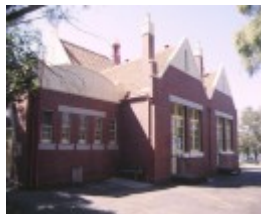
infant building & shelter shed coburg primary school no 484 bell street coburg side view feb 98
