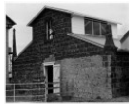
Warrawong Shearing Shed
