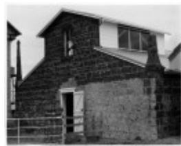
Warrawong Shearing Shed
