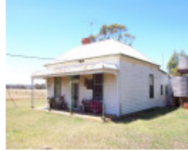
Late Victorian era dwelling on the property
