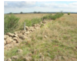
Dry Stone Wall K166 - south boundary
