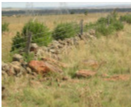
Dry Stone Wall K165 - north boundary
