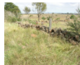
Dry Stone Wall K164 - Eastern Boundary
