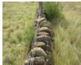
Dry Stone Wall K164 - Eastern Boundary
