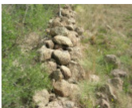
Dry Stone Wall K166 - south boundary
