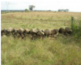
Dry Stone Wall K164 - Eastern Boundary
