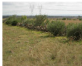
Dry Stone Wall K166 - south boundary
