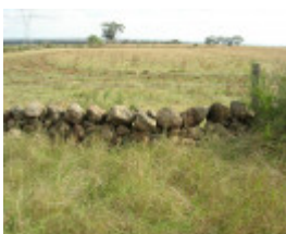
Dry Stone Wall K164 - Eastern Boundary
