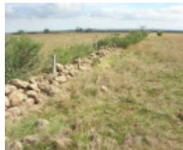
Dry Stone Wall K166 - south boundary
