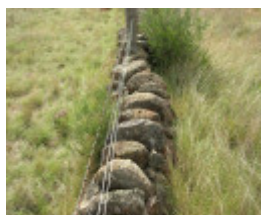
Dry Stone Wall K164 - Eastern Boundary
