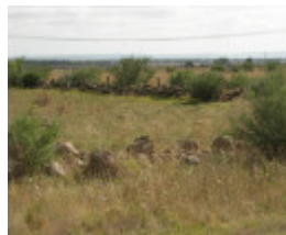
Dry Stone Wall K166 - south boundary
