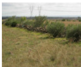
Dry Stone Wall K166 - south boundary
