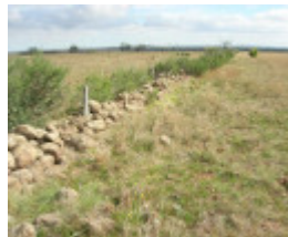
Dry Stone Wall K166 - south boundary
