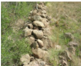
Dry Stone Wall K166 - south boundary
