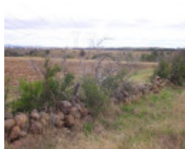
Dry Stone Wall K165 - north boundary
