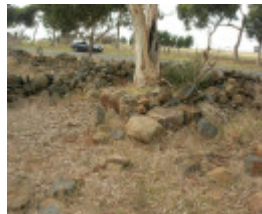
Dry Stone Wall K159 - eastern boundary
