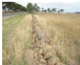
Dry Stone Wall K159 - eastern boundary
