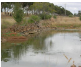
Dry Stone Wall K159 - eastern boundary
