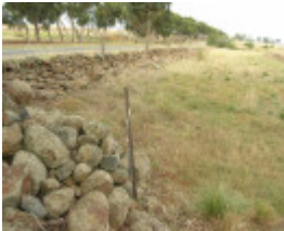
Dry Stone Wall K159 - eastern boundary
