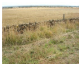
Dry Stone Wall K159 - eastern boundary
