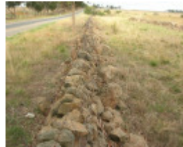
Dry Stone Wall K159 - eastern boundary
