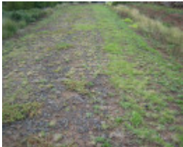
Rockbank Middle Road pavement
