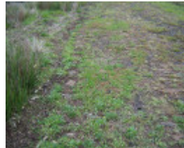
Rockbank Middle Road pavement
