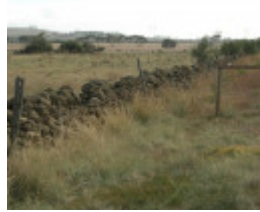
Dry Stone Wall F181 - western boundary
