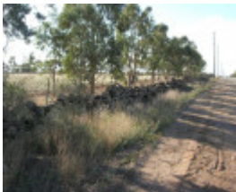
Dry Stone Wall F186 - southern boundary
