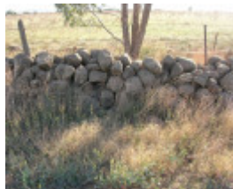
Dry Stone Wall F186 - southern boundary
