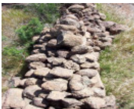
Dry Stone Wall F94 - eastern boundary
