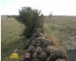
Dry Stone Wall F181 - western boundary
