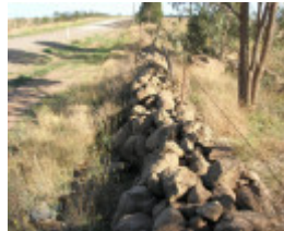
Dry Stone Wall F186 - southern boundary
