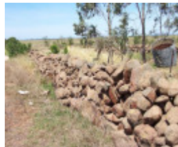
Dry Stone Wall F94 - eastern boundary
