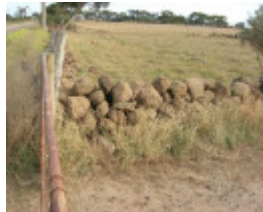
Dry Stone Wall F181 - western boundary
