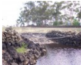
Dry stone wall dam, with cobbled ramp
