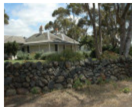
Dry Stone Wall B28
