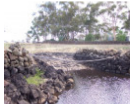
Dry stone wall dam, with cobbled ramp
