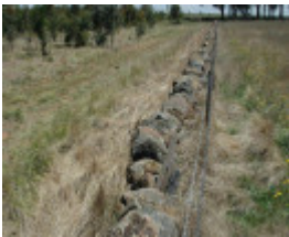
Dry Stone Wall B76
