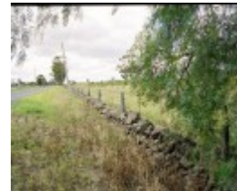
Dry Stone Wall B127 - eastern boundary
