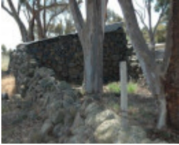
Dry Stone Wall B75
