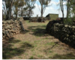
Dry Stone Wall B75
