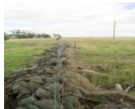
Dry Stone Wall B129 - northern boundary
