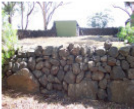
Dry stone wall stock yard
