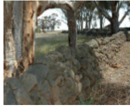
Dry Stone Wall B75
