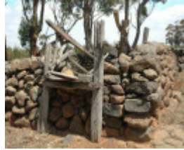
Dry Stone Wall B75
