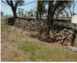
Dry Stone Wall B74
