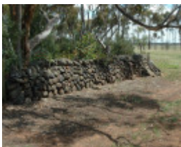
Dry Stone Wall B28
