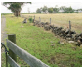
Dry Stone Wall B128 - southern boundary
