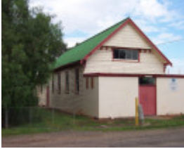
Rockbank Community Hall
