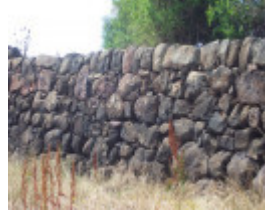
Rockbank Headstation Dam Wall
