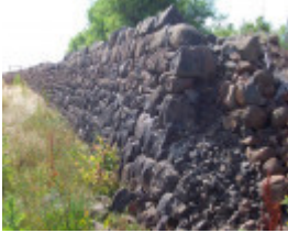
Rockbank Headstation Dam Wall
