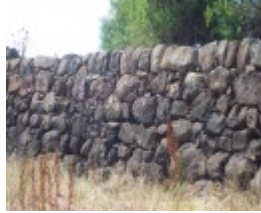
Rockbank Headstation Dam Wall
