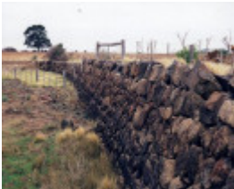
Dry Stone Wall N238 - Rockbank Headstation Dam Wall
