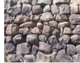
Rockbank Headstation Dam Wall - detail
