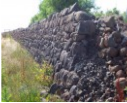
Rockbank Headstation Dam Wall
