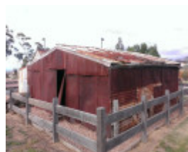
Dairy Buildings - May 2013
