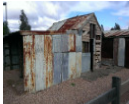
Dairy Buildings - May 2013
