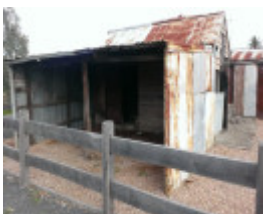
Dairy Buildings - May 2013
