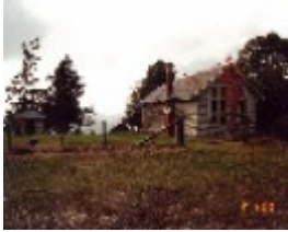
Arawata State School No. 2970 (former)
