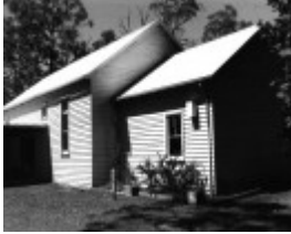
Pakenham Upper Civic & Residential Precinct & Upper hall
