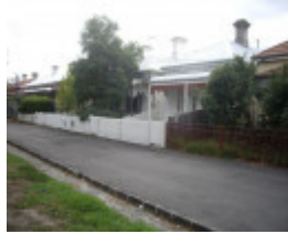
HO7(2) - Old Footscray Township Residential Area.JPG
