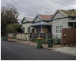
HO15(1) - Yarraville Residential Heritage Area.JPG
