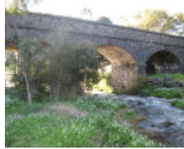
H1446 Newlands Road Bridge 3 Sep 2008
