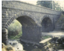
bridge newlands road coburg side detail
