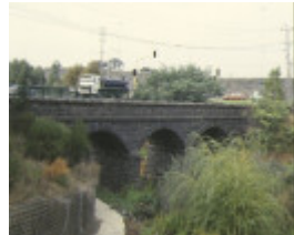
bridge newlands road coburg side view
