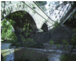
bridge newlands road coburg side elevation sep1984
