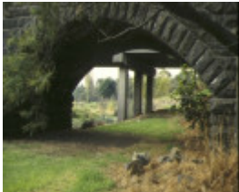
bridge newlands road coburg detail of arch may1997
