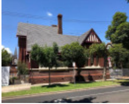
9-23 Densham Road, Armada
