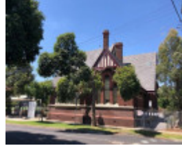
9-23 Densham Road, Armada
