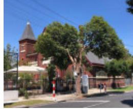
9-23 Densham Road, Armada
