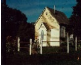
Dumbalk North Methodist Church (former)
