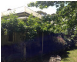
Greenfields south gable
