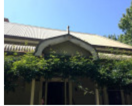
Greenfields verandah gablet
