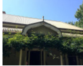
Greenfields verandah gablet
