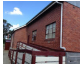
Fish Creek Memorial Hall 1959 Supper Room addition
