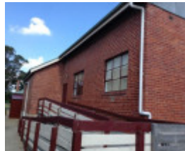
Fish Creek Memorial Hall 1959 Supper Room addition
