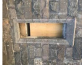
Repairs to B1
