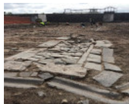
Pentridge excavation by Dig Intl
