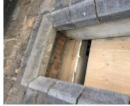
Repairs to B1
