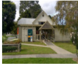
Former Court House
