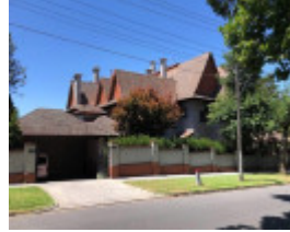
224 Kooyong Road, Toorak
