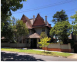
224 Kooyong Road, Toorak
