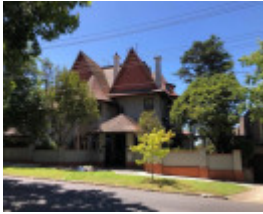
224 Kooyong Road, Toorak
