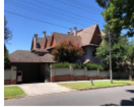
224 Kooyong Road, Toorak
