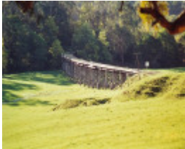
Three Railway Bridges
