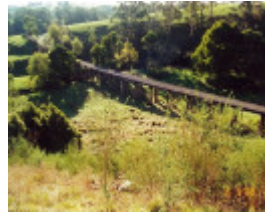
Three Railway Bridges
