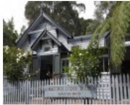
Former Kilcunda Road State School
