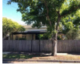
66-72 Peel Street, Windsor
