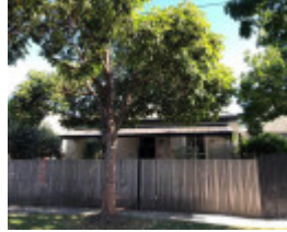
66-72 Peel Street, Windsor
