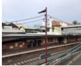
Malvern Railway Station
