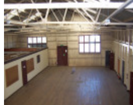
Drill Hall internal prior to conversion to sport facility
