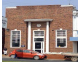
CBC Bank (former, 2020)
