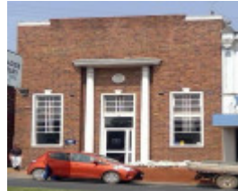
CBC Bank (former, 2020)
