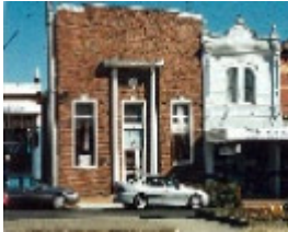
CBC Bank (former, 2000)
