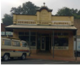
Falconer Building (former, 2020)
