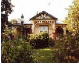
Dwelling at 20 Victoria Street Korumburra 3950
