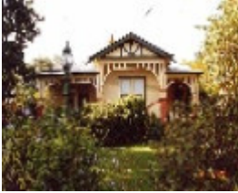
Dwelling at 20 Victoria Street Korumburra 3950
