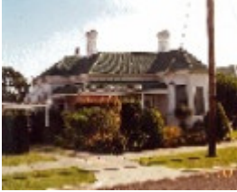
Dwelling AT 25 Victoria Street Korumburra 3950
