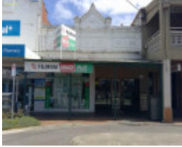
Shops, 8-10 Bair Street (2020)
