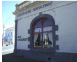
former adam reas store colac detail side window feb1985
