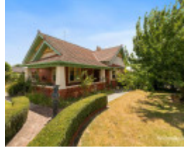
House, 45-47 Roughead St
